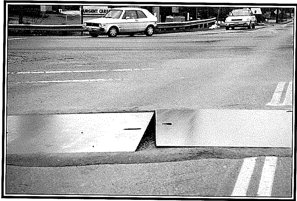
It's a good idea to stay away from the edges of steel construction plates.
